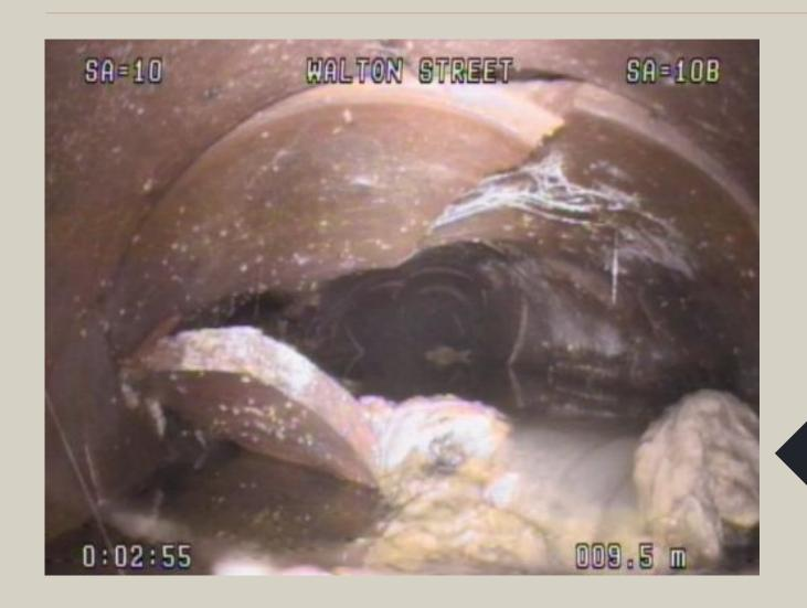
Multiple aging clay and brick sanitary sewers, circa 1920s, collapsing. Some of which were previously combined storm/ sanitary sewers
