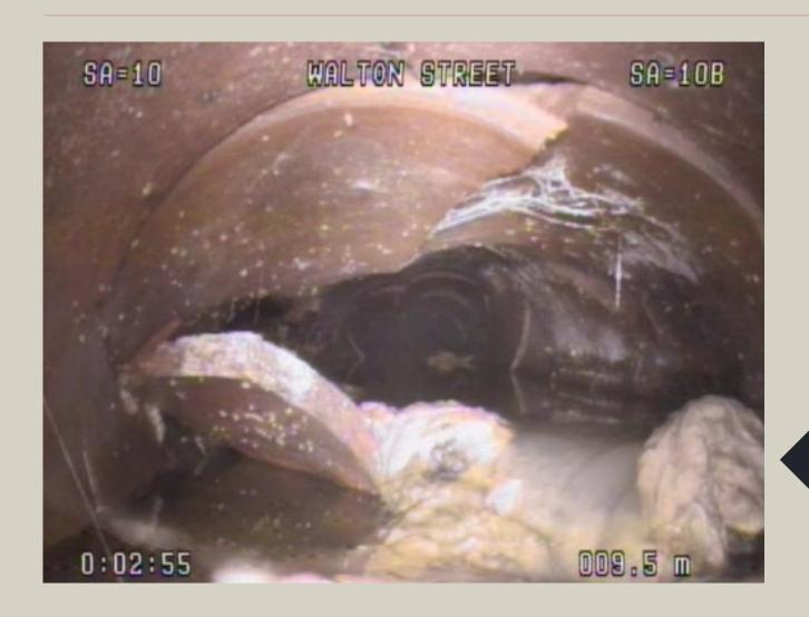
Multiple aging clay and brick sanitary sewers, circa 1920s, collapsing. Some of which were previously combined storm/ sanitary sewers
