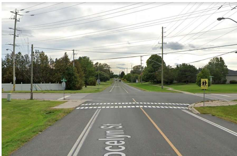
Figure 2-6: Jocelyn St, Facing West (Google, September 2021)
